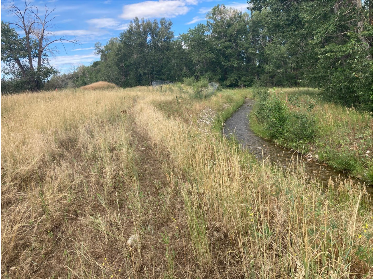
Figure 3. Desert Canal, seen looking west from near the existing concrete head gate. Cobble slope between upland and canal bank is visible near the center of the photo; browsing exclosures are also visible in the distance.
